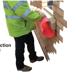
Coping Cramp and Dowel Refer to technical installation instructions
